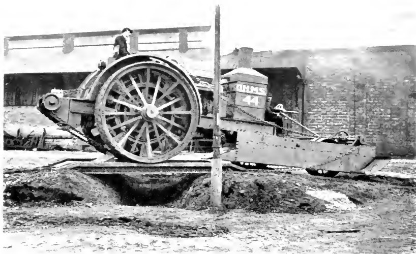
TRITTON'S TRENCH CROSSING MACHINE. (p. 30)
