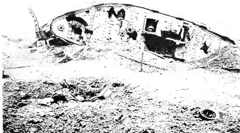
TANKS OUT OF ACTION ( p. 195 )
