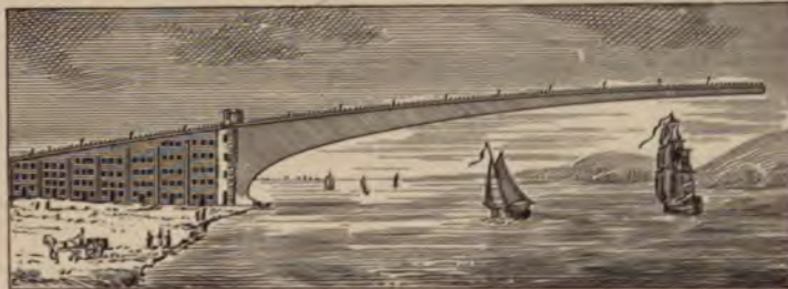
Pope's Cantilever in Process of Erection. (From his "Treatise on Bridge Architecture.")
