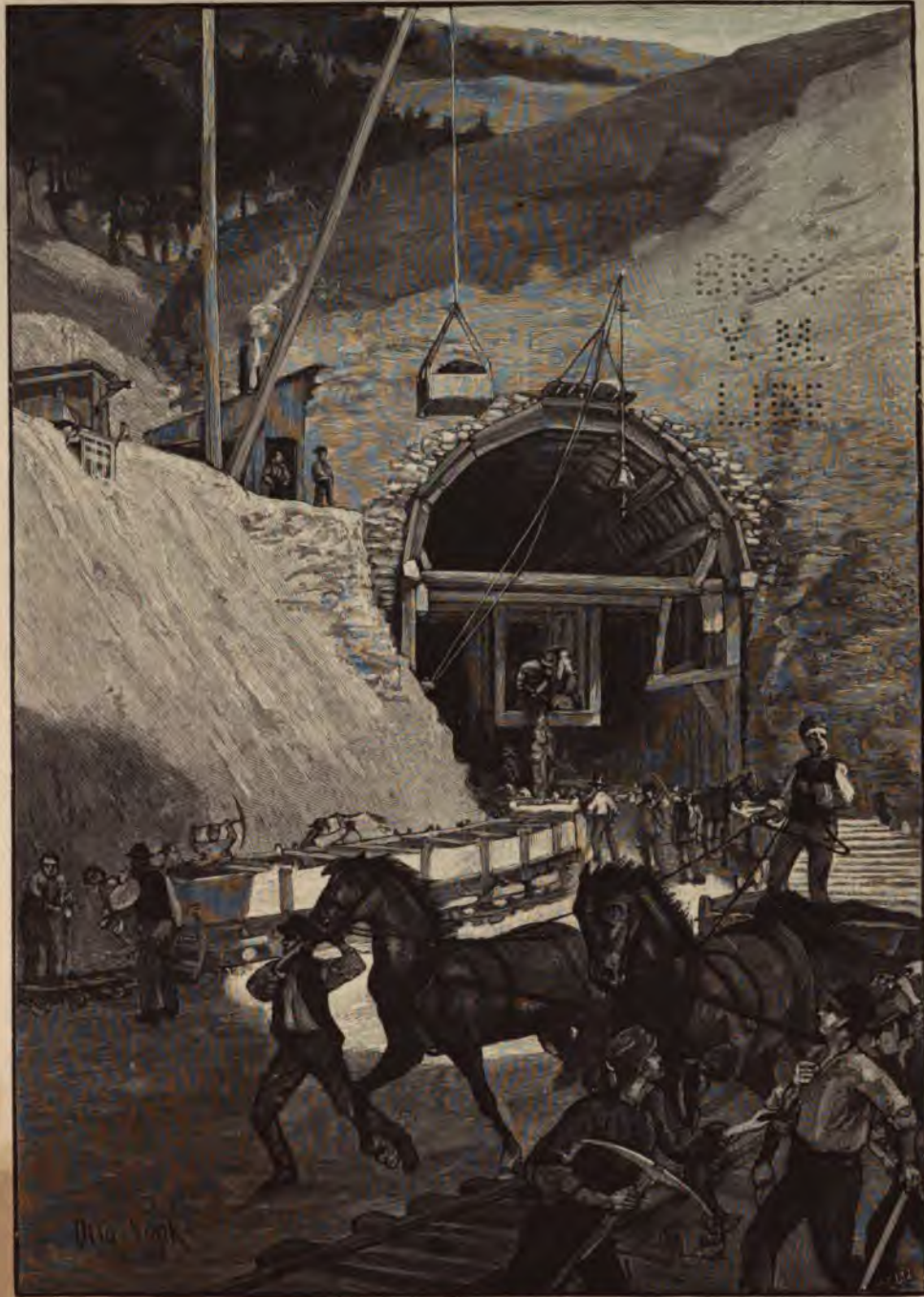
Portal of a Tunnel in Process of Construction.
