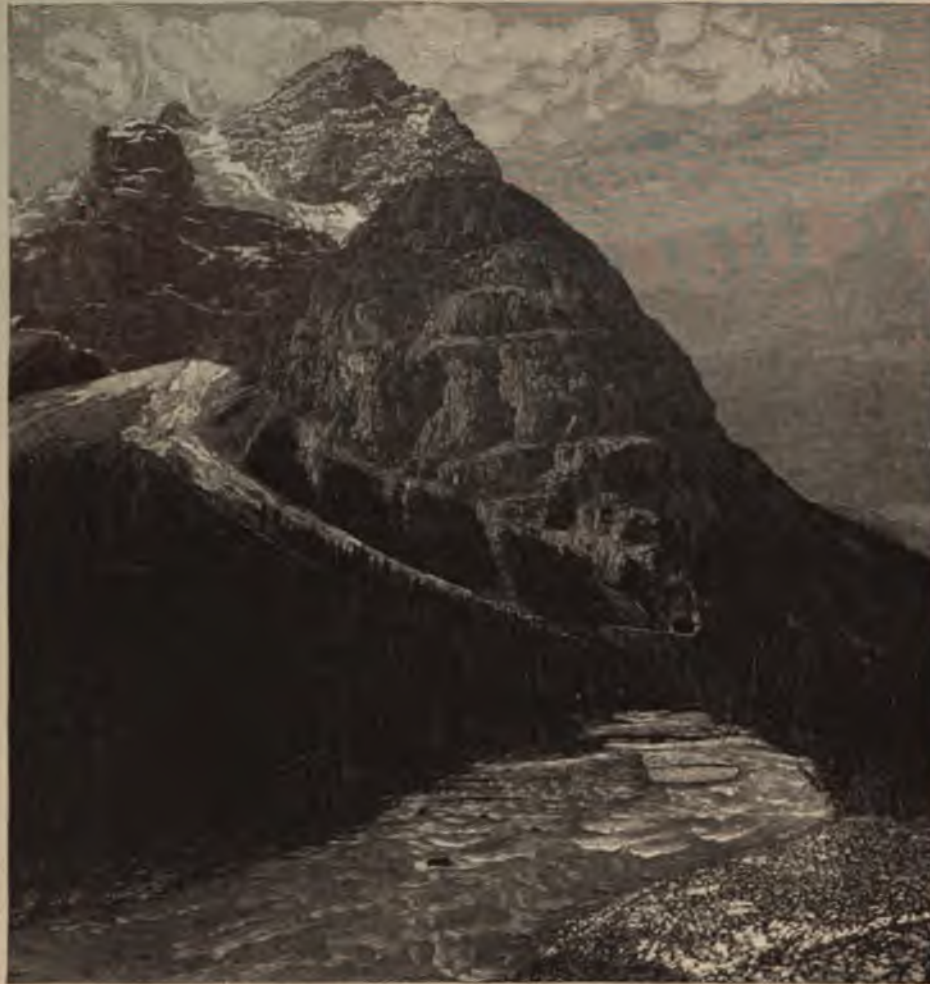
Tunnel at the Foot of Mount St. Stephen, on the Canadian Pacific. (The glacier 8,200 feet above the Railway.)
