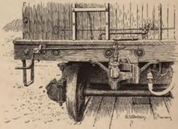
Janney Automatic Coupler applied to a Freight Car.
