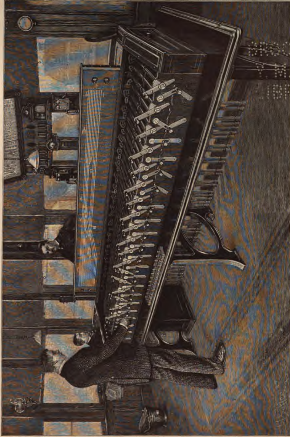
Interlocking Apparatus for Operating Switches and Signals by Compressed Air, Pittsburg Yards, Pennsylvania Railroad. (A model of the track is shown above the levers, on which the movements of the switches and signals are electrically indicated after they are completed.)
