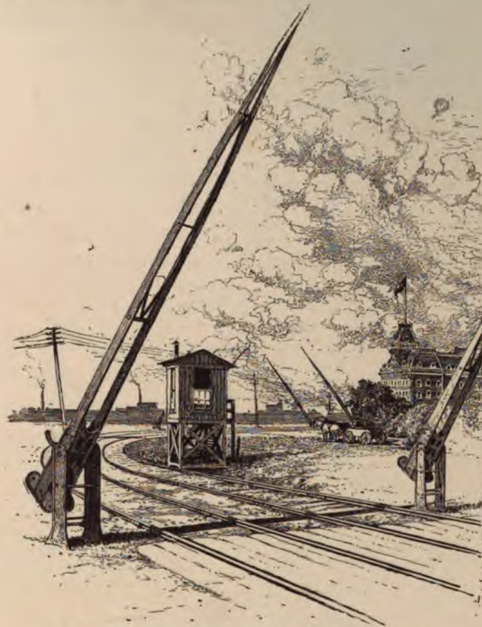
Crossing Gates worked by Mechanical Connection from the Cabin.
