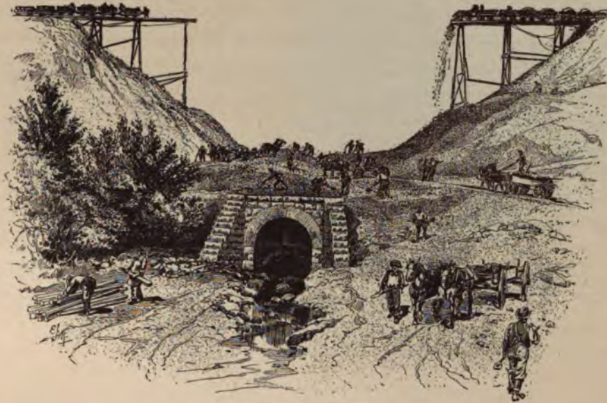
Making an Embankment.
