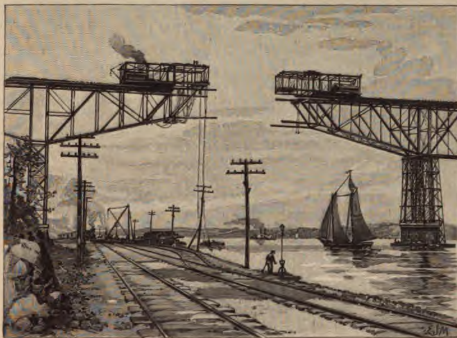
Erection of a Cantilever.
