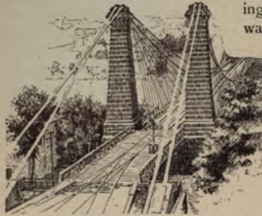
Old Stone Towers of the Niagara Suspension Bridge.
