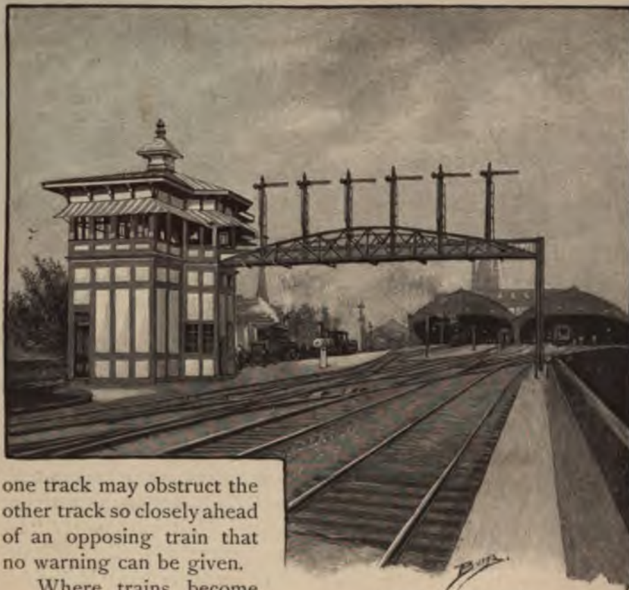
Central Switch and Signal Tower.
