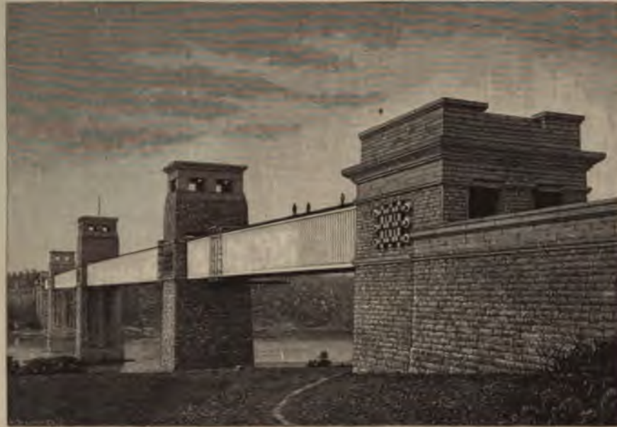
The Britannia Tubular Bridge over the Menai Straits, North Wales.
