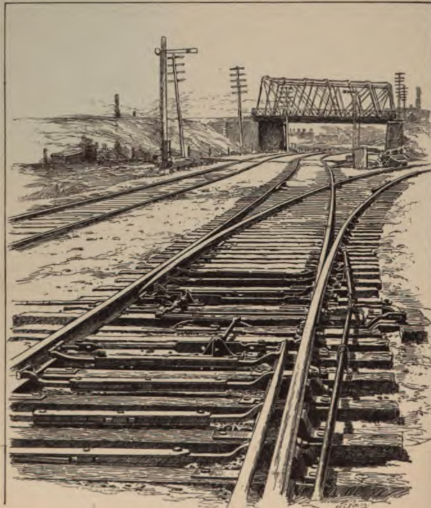
Split Switches with Facing-point Locks and Detector-bars.
