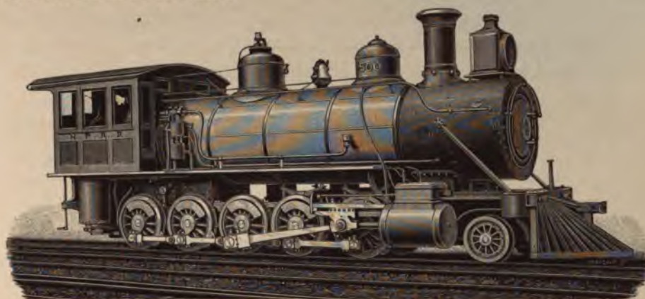
Fig. 31.—Decapod Locomotive. By the Baldwin Locomotive Works, Philadelphia.
