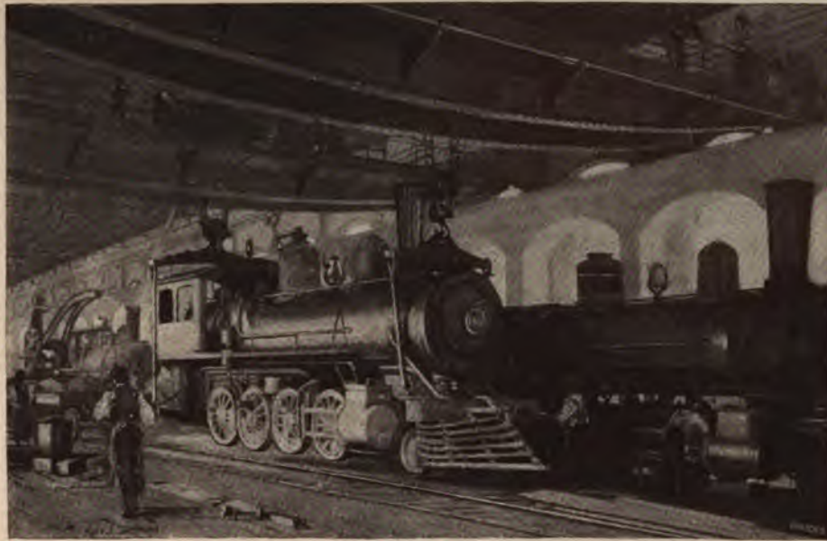
Fig. 38.—Interior of Erecting Shop, Showing Locomotive Lifted by Travelling Crane.
