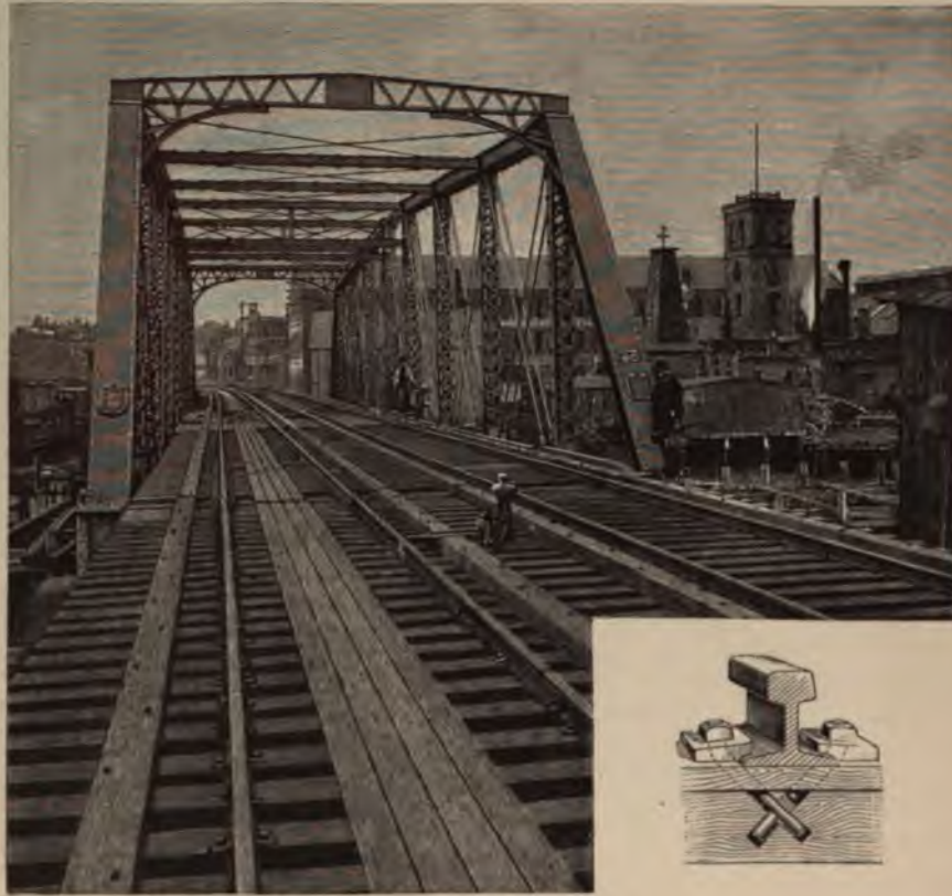
New South Norwalk Drawbridge. Rails held by safety bolts.
