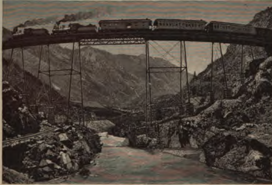
Curved Viaduct, Georgetown, Col.; the Union Pacific crossing its own Line.
