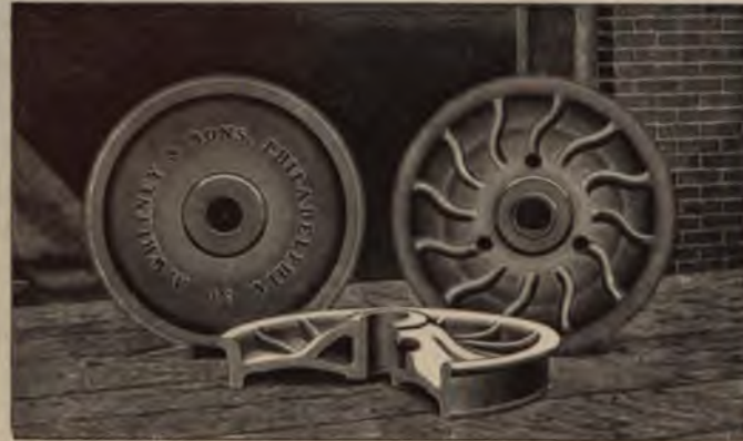
Fig. 51.—Cast-iron Car Wheels.
