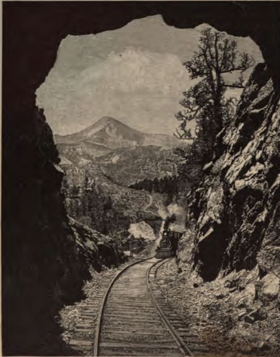
Portal of a Finished Tunnel; showing Cameron's Cone, Colorado.
