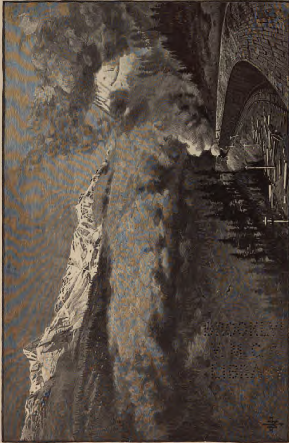
Snow-sheds, Selkirk Mountains, Canadian Pacific. The winter track under cover; the outer track for summer use.
