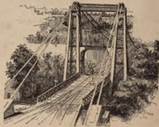
The New Iron Towers of the Same.
