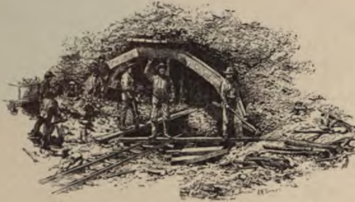
Beginning a Tunnel.
