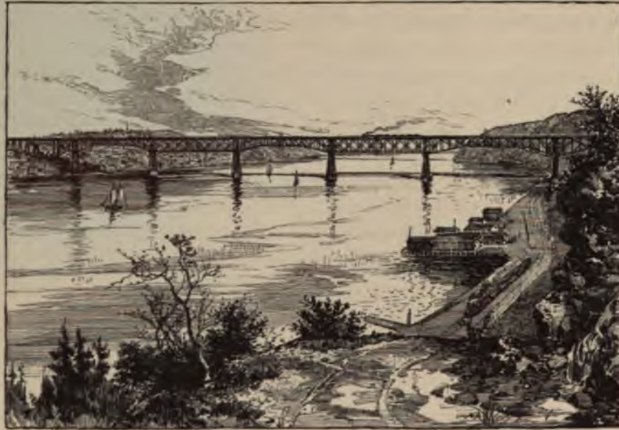
General View of the Poughkeepsie Bridge.
