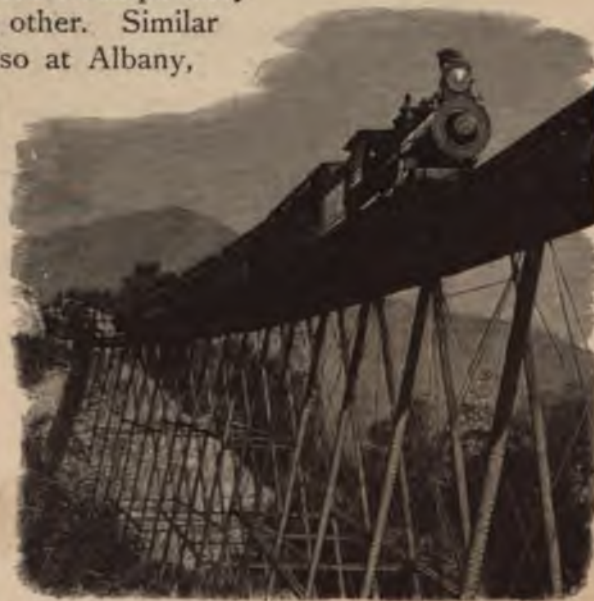
Trestle on Portland and Ogdensburg Railway, Crawford Notch, White Mountains.
