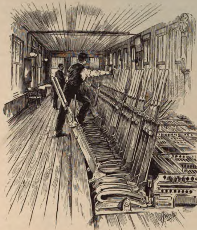
Interior of a Switch-tower, showing the Operation of Interlocking Switches.
